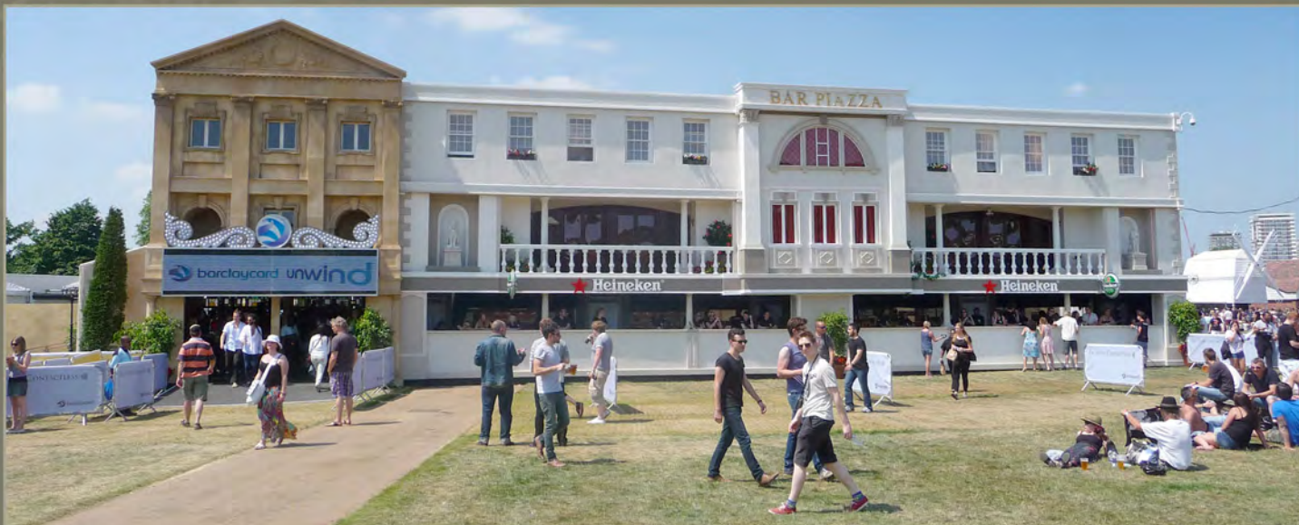
Three storey bar and venue entrance built from nine shipping containers at Hyde Park British Summer Time Festival.
